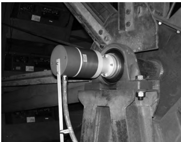
Fig. 11. New slip ring unit during testing period in 2006. Courtesy of ZKM.
