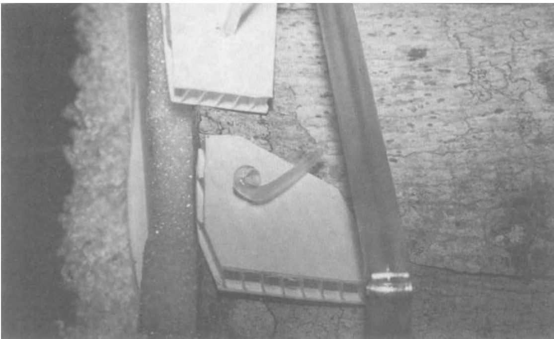
Figure 5. The polypropylene rod pin is heated locally and curled to make a head.
