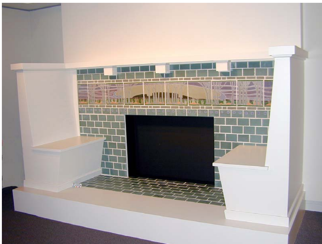
Figure 15. Panels installed with surround.
